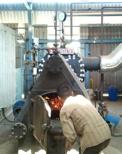
Solid Fired Membrane Type SIB Boiler
